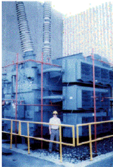
PJM Public Service Step Up Transformer Severe internal damage caused by the space storm of 13 March, 1889.
