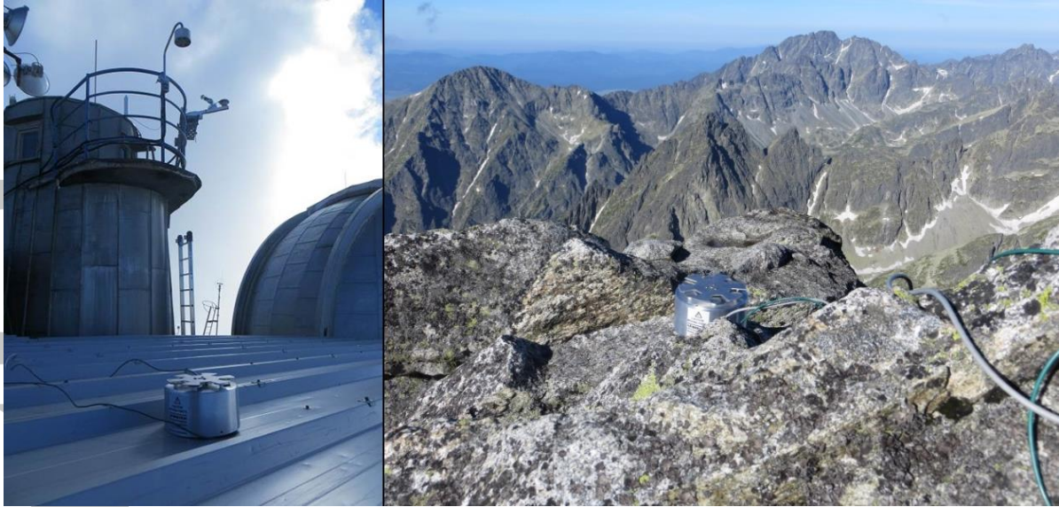
Fig. 1. Left: the installed EFM in inverted position (fixed to the fence in the upper part of Figure) and the reference EFM during calibration (in the front part). Right: the reference EFM during calibration at one of the locations used for calibration.
