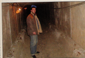
Where the sun doesn't shine. In winter, underground tunnels are often the only way for technician Tigran Yepisposian and others to move between buildings.
