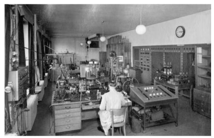
Laboratory of the Max Planck Institut für Instrumentenkunde in 1948, where Heinz Billing invented the first magnetic storage system for computers. The institute was founded in 1946 to develop new scientific apparatuses, which would enable other institutes to start new projects or improve their ongoing research with more effective devices.
