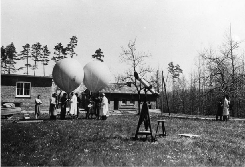
ILLUSTRATION 71 Research Center for Stratospheric Physics, Weissenau, early post-war years. Preparing the launch of a Regener's balloon tandem. The telescope was used to track the balloon tandem so that the payload could potentially be recovered intact before it touched the ground.
