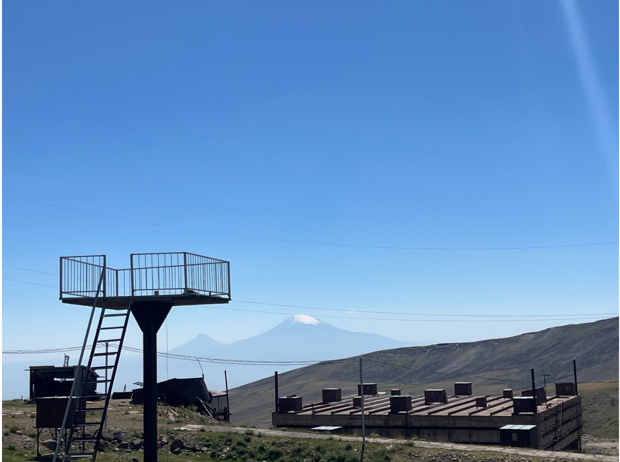
Figure 8. A new platform prepared by CRD for installing particle detectors, panoramic cameras, near-surface electric field sensors, and weather stations. CRD will provide electricity, internet, and maintenance for groups worldwide planning advanced experiments in cosmic rays, atmospheric physics, and Space weather.
