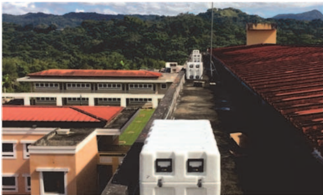
Figure 5. Four of 10 TETRA-II detector boxes on roof of Building B, UPR-Utuado.
